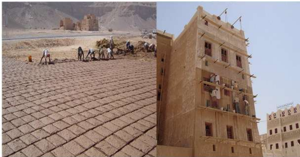
Figure 6: Labourers Preparing of Clay Bricks by Traditional Methods and Skills of Builders in Constructing Buildings.
