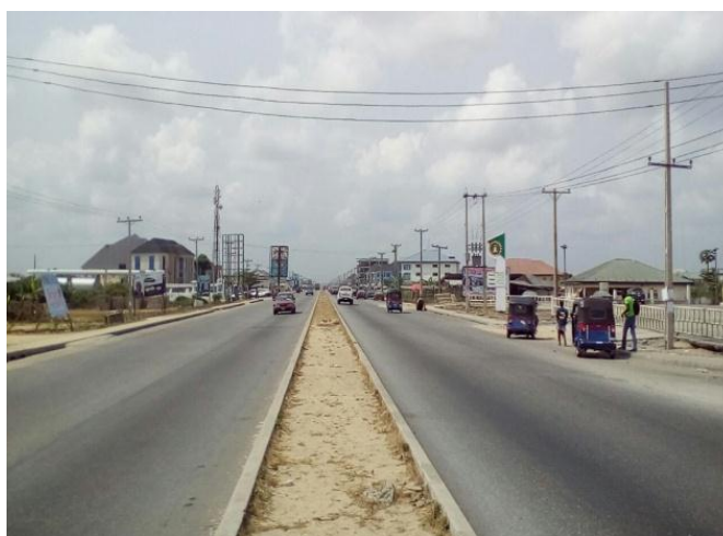
Fig. 11: Isaac Adaka Boro Road without Drainage in the Study Area.
