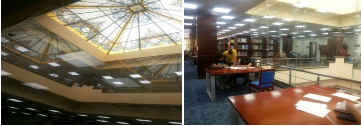
Figure 13: BUE library building- Atrium covered by skylight to maximize natural lighting entering the reading space.
