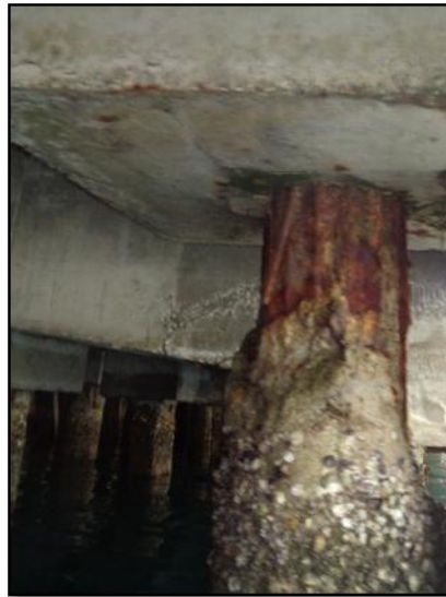
Figure 1: Photo of Corroded Reinforced Concrete Pile.
